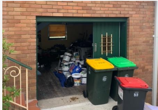
Figure 6 – View North towards the existing attached single garage
