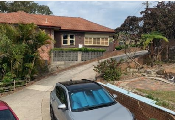
Figure 5 - View east towards the existing retaining wall, driveway, and 47 Homer Street from the front of the existing dwelling
